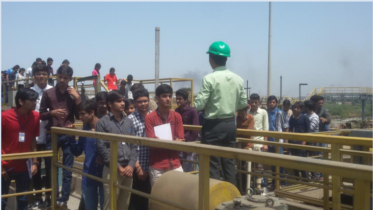
Image: Secondary Treatment Plant
