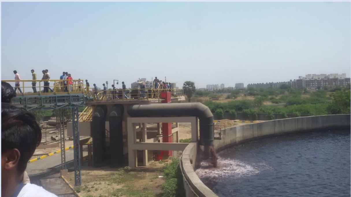
Image: Removal of west Sludge from water by Clarifying Filter
