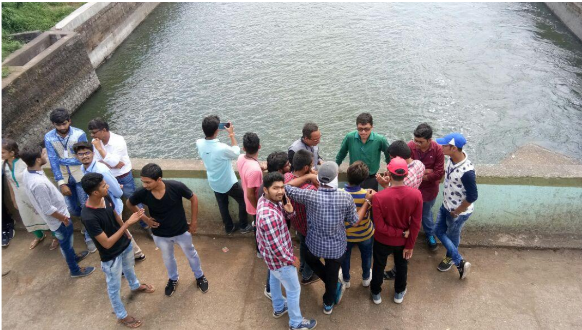
Figure 3: Kakrapar Main Canal
