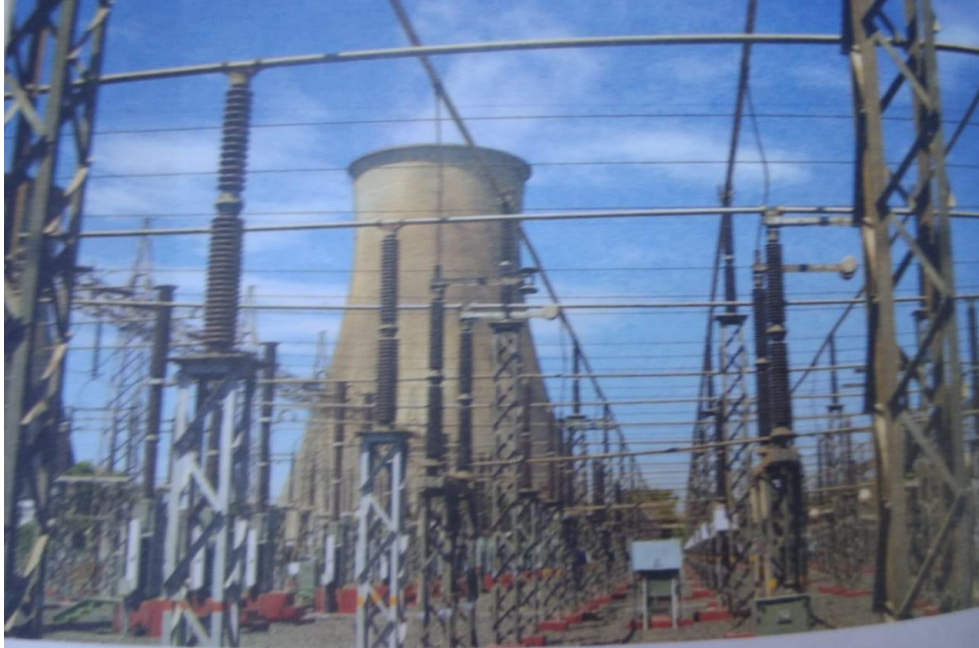
Electricity Generation System, NPCIL, Kakrapar
